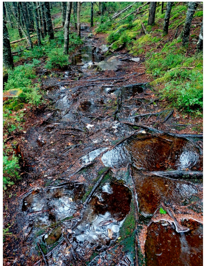
Fig. 7. Incised contour-aligned (flat) side-hill trails collect and retain water after rains and can be difficult to keep drained.
